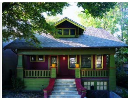
Garden-variety Arts & Crafts porches like this bungalow's were lean on millwork compared with Victorian houses, but railings and piers were regularly ordered from catalogs—often along with the rest of the building. (Photo: Doug Keister)
