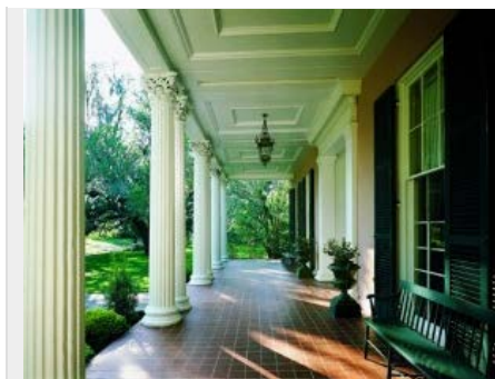
In keeping with temple models, the porticos on high-style classical houses often eschewed railings while making the most of other millwork details, such as the fluted columns and paneled ceiling seen here. (Photo: Paul Rocheleau)
