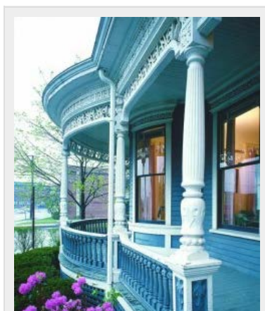
Typical of Victorian houses at their peak, this porch is supported by slender turned posts with machine-carved decoration covering the entire surface. Similar-looking balusters help integrate the wealth of complicated ornament. (Photo: Brian Vanden Brink)
