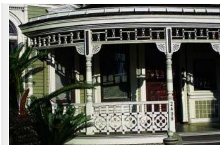
By 1870, balusters fret-sawn from flat boards were common millwork items, along with turned spandrels that bridged the tops of many porches with "Steamboat Gothic" ornament. (Photo: Ken Naversen)
